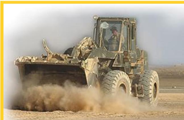
**KEEP 'EM FLYING** Every morning the "pulverized" face of Rhino's runway was scraped away. (Photo courtesy of US Navy/Photographer's Mate First Class Greg Messier )
